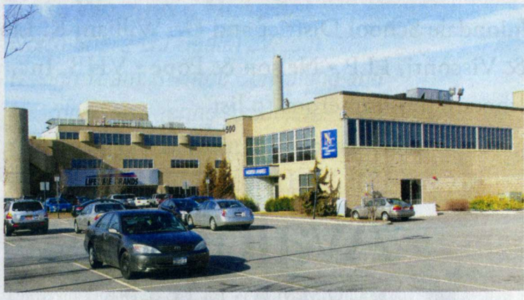
1000 Stewart Ave. and 500 Endo Blvd.
